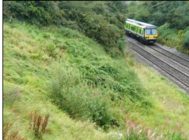
Plate 3.2 – Railway embankment in Kildare (Photo: M. Tubridy).
